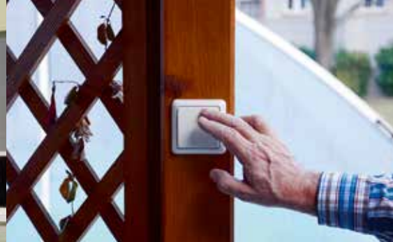
Wireless switching in gardens
